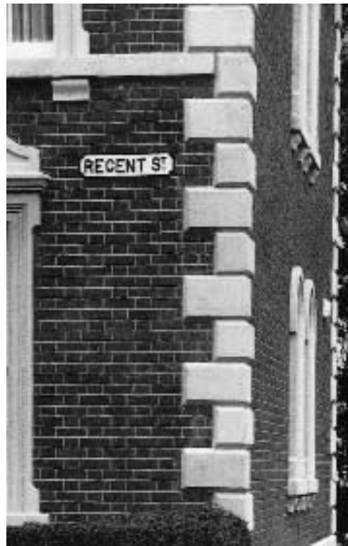
Figure 3.1 Quoined corner, Regent Street, Nottingham
